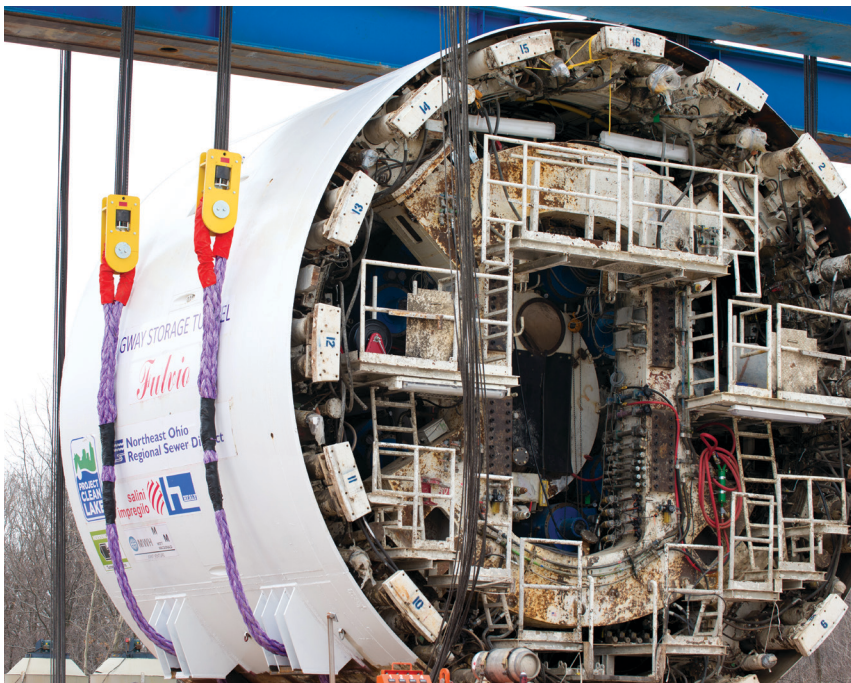
Cortland's Plasma® 12x12 lifting slings around the 495-tonne boring machine
