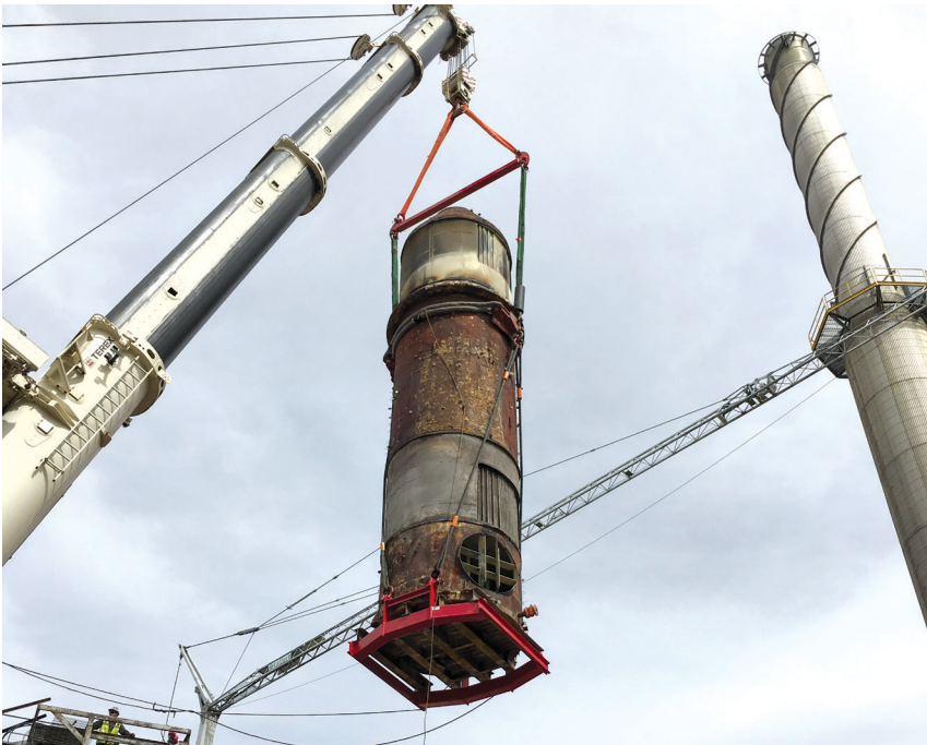
The heat exchanger during vertical lift, showing red basket frame and sling to support the aging structure.
