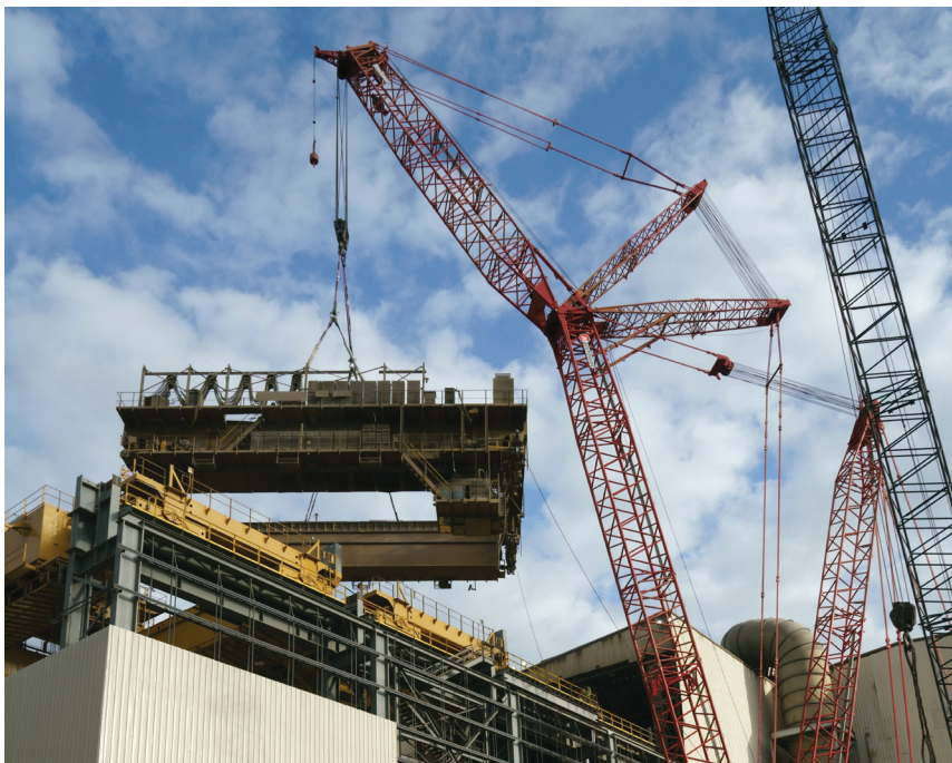
Removal of one section of 300 ton bridge crane
