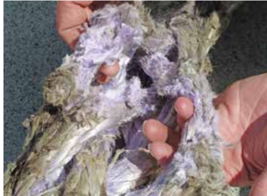
Excessive interior abrasion wear
