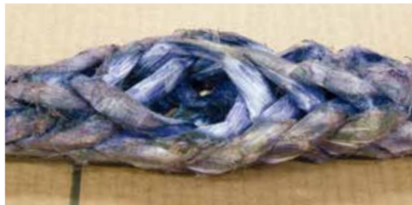
Example of moderate external damage but minimal internal damage
